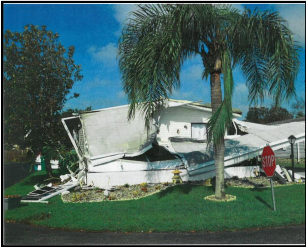
Older carport damage and screen room damage. All homes stayed on their foundations.
