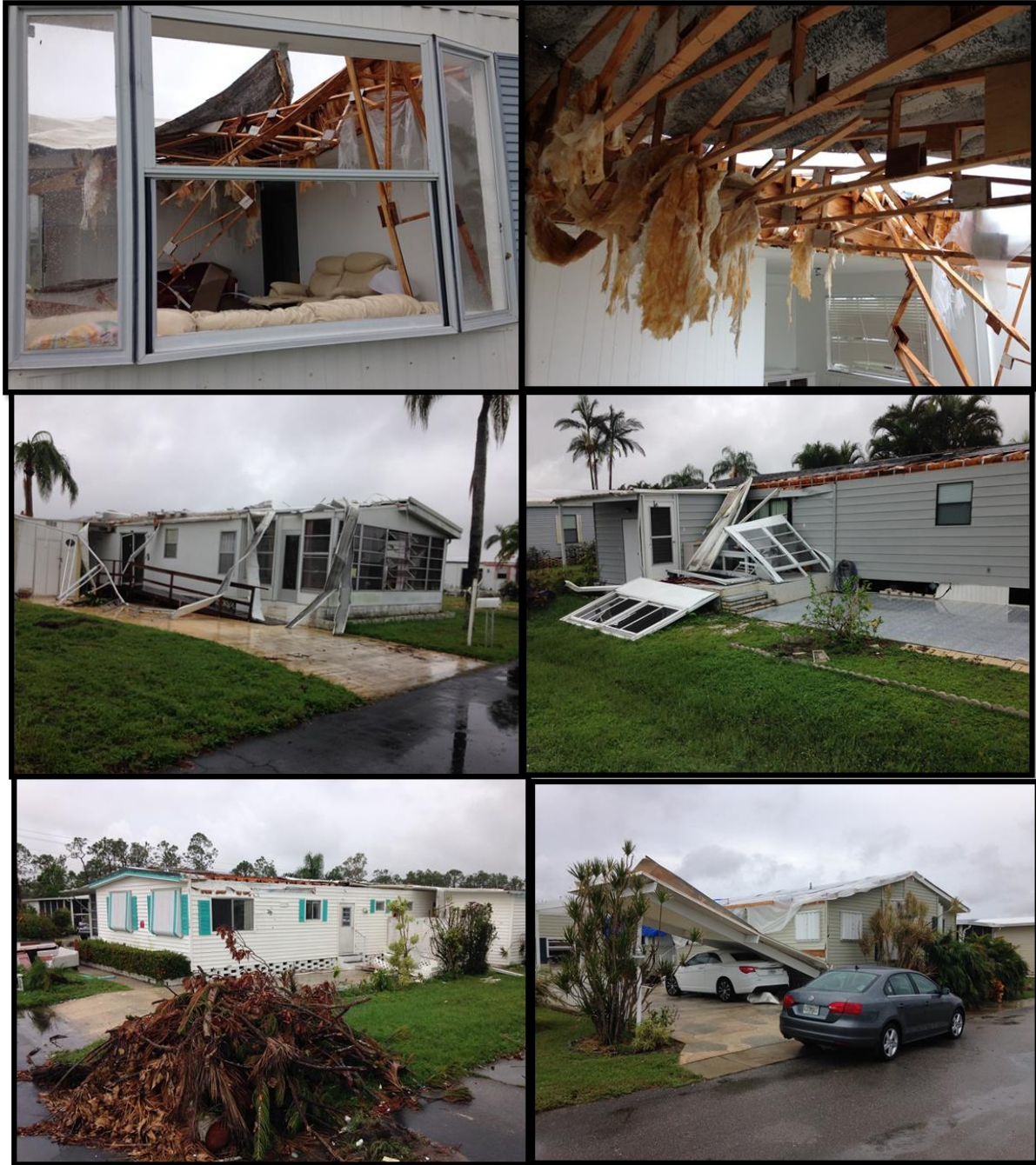
Naples - older manufactured homes with lighter weight carport damage causing extensive damage to the homes.
