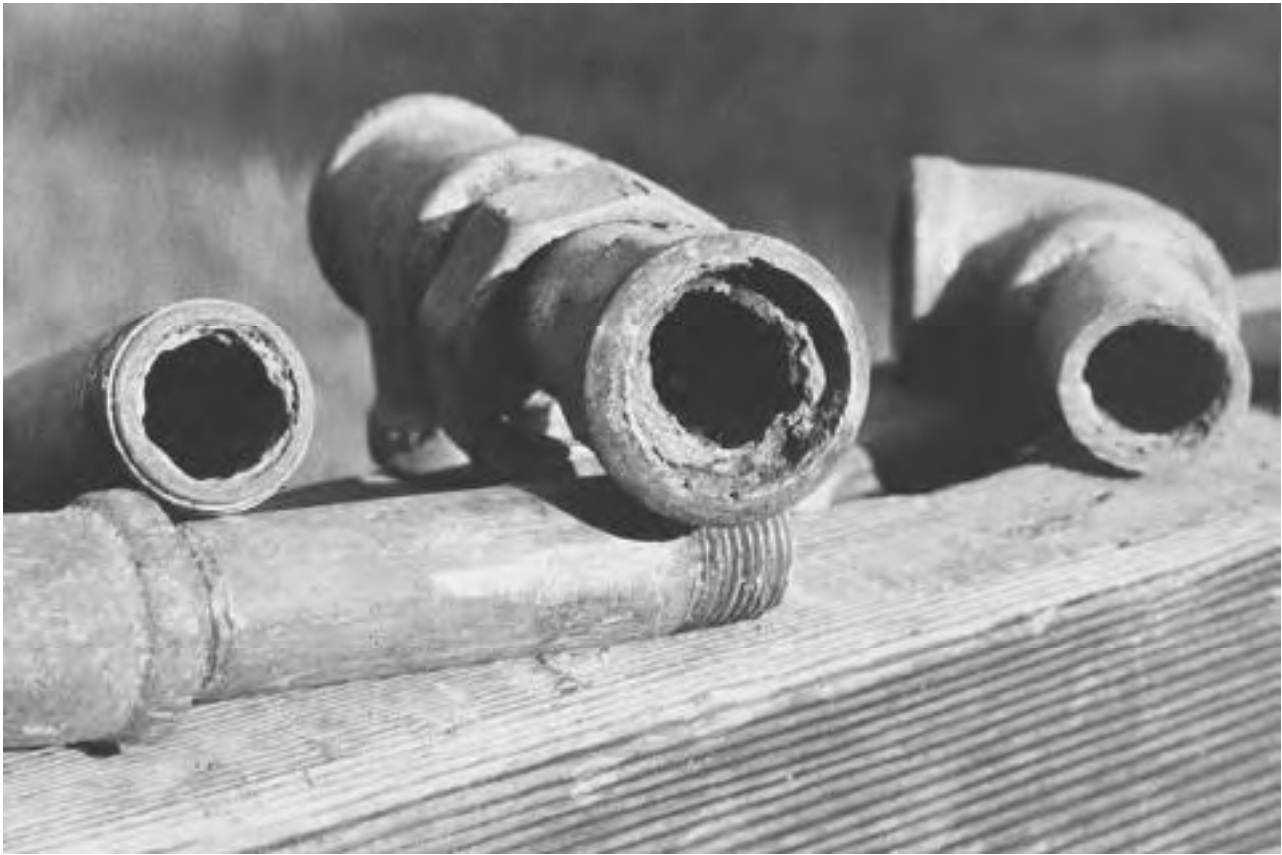
Galvanized pipe sections removed from an older house. Mineral deposits and corrosion within the pipe had severely reduced water flow to the plumbing fixtures.
