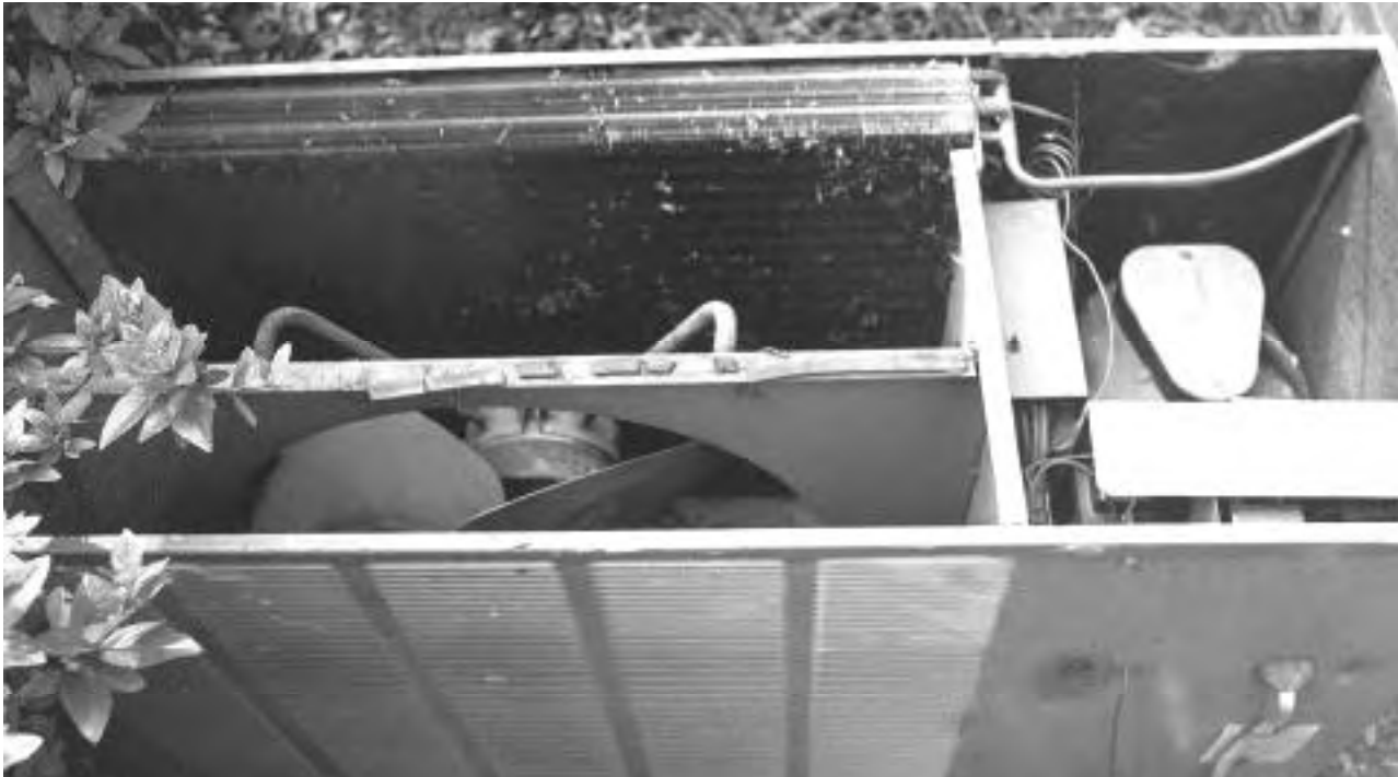
Looking down into an outdoor compressor unit with the top cover removed. The compressor is on the upper right, controls are on the lower right, and the fan and condenser coils are to the left.
