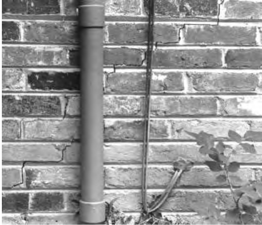
A common masonry wall crack probably caused by thermal or moisture expansion. If possible, monitor such cracks over a period of time to see if they're active. Active cracks should be sealed with a flexible sealant; inactive cracks may be painted.
