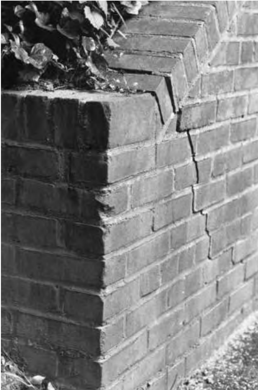
The outward movement of the upper part of this retaining wall can be halted only by structural reinforcement. Simply patching the crack will not solve the problem.
