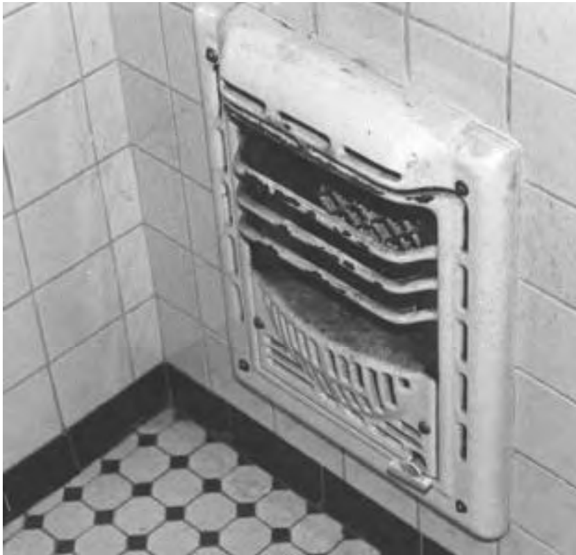
Check the heating source in every room. This particular heater, when tested, was operable and safe.
