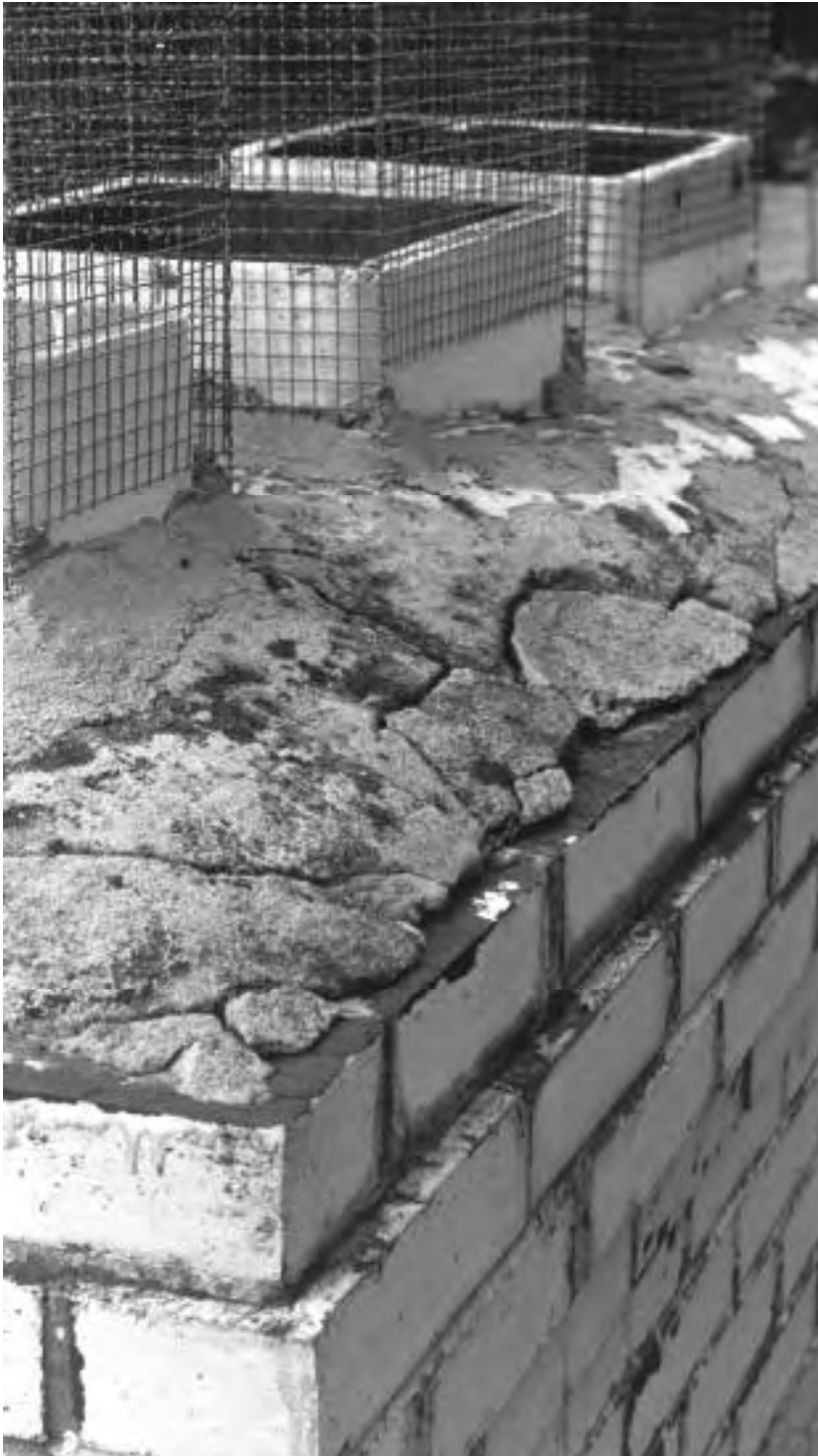
A deteriorated chimney cap. Mortar, rather than concrete, is often improperly used (as it was here) to cap the chimney. The masonry below will eventually deteriorate unless the cap is replaced.
