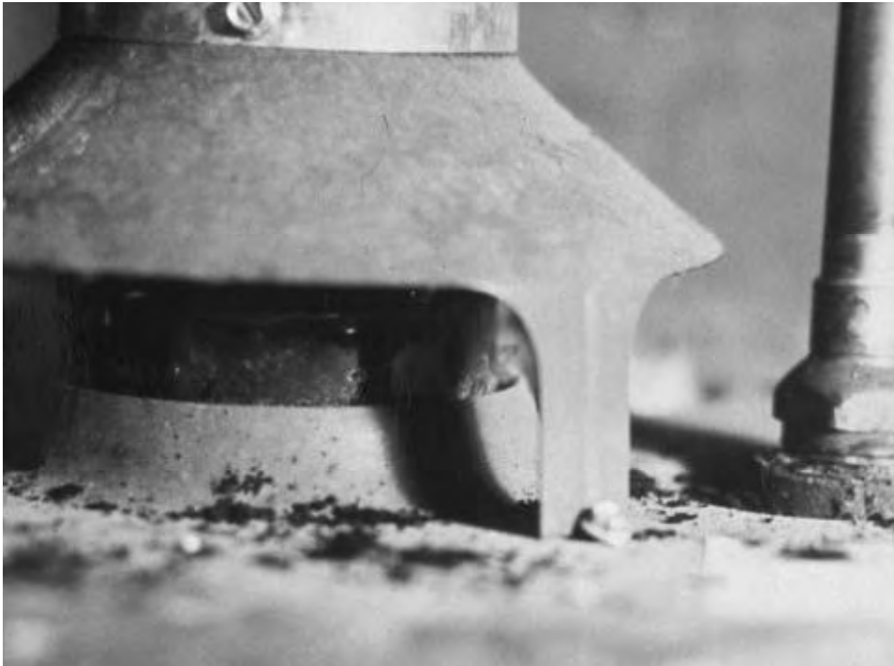
The soot that has accumulated below the draft hood of this water heater indicates a severely clogged flue or chimney, or more commonly, back-drafting caused by insufficient make-up air.
