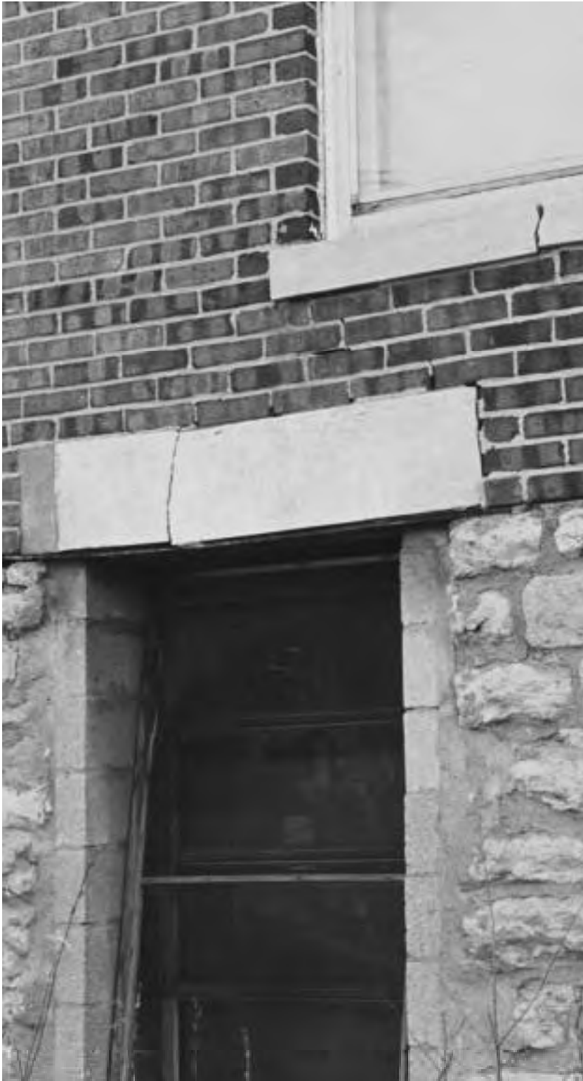
Failure of a concrete lintel and sill due to differential settlement of the building. Permanent repairs will be quite expensive. Note the makeshift shoring of the lintel.
