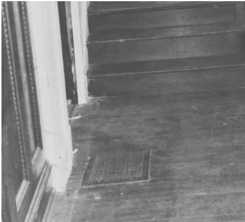
The sagging floor is caused by settlement of a basement support. It may be possible to jack the floor and its adjacent wall into a level position, but this should be done slowly and carefully.
