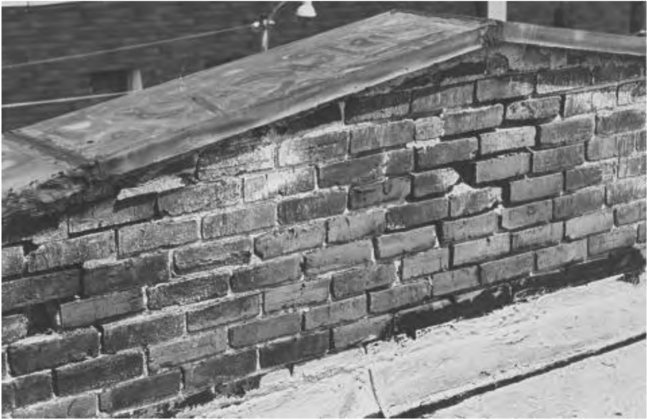
A deteriorated parapet wall that badly needs repointing. Fortunately, the wall has not yet exhibited serious movement, but it will if left unrepaired.
