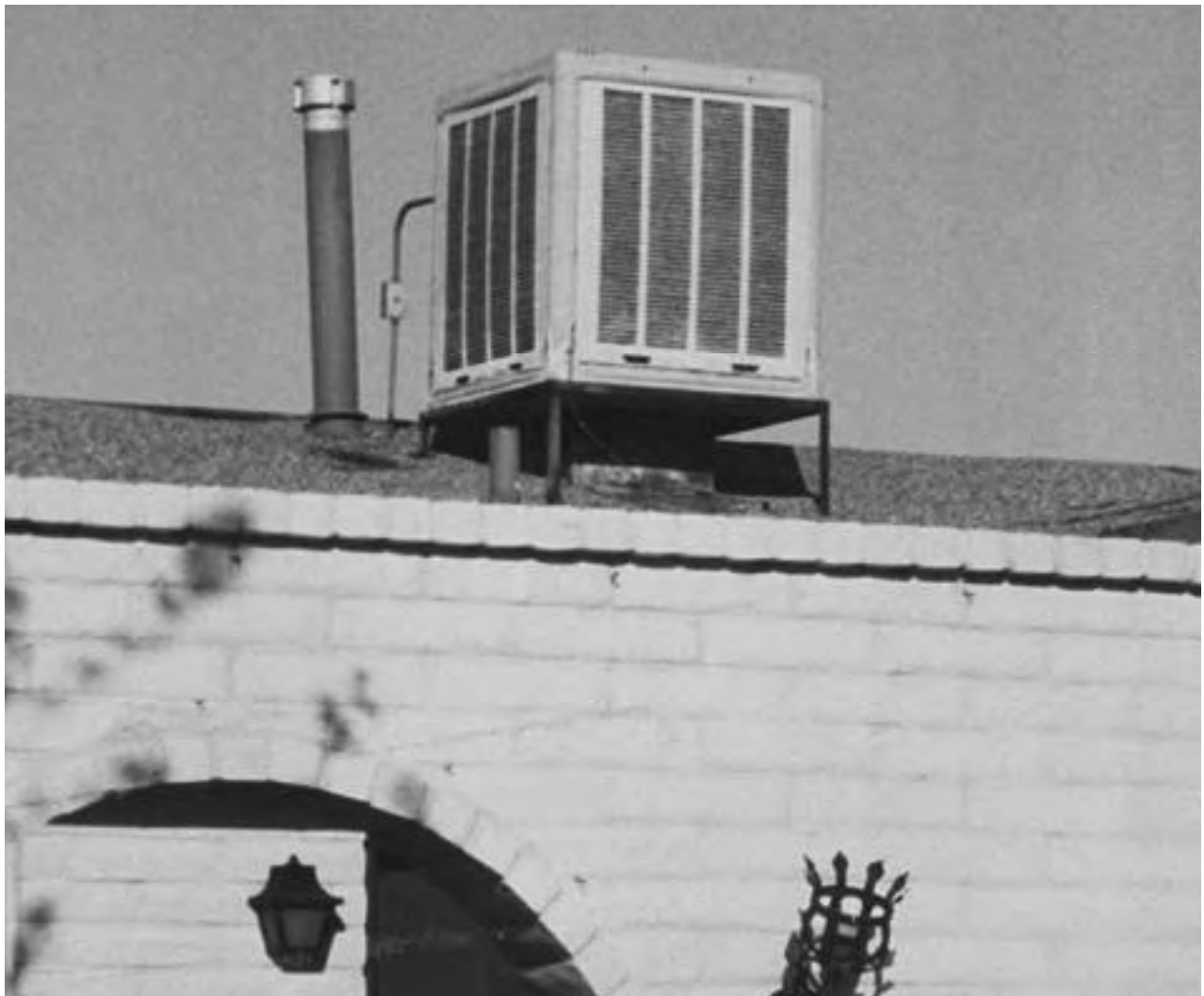
A roof-mounted evaporative cooler. This type of cooling unit is relatively simple to inspect, repair, and maintain.
