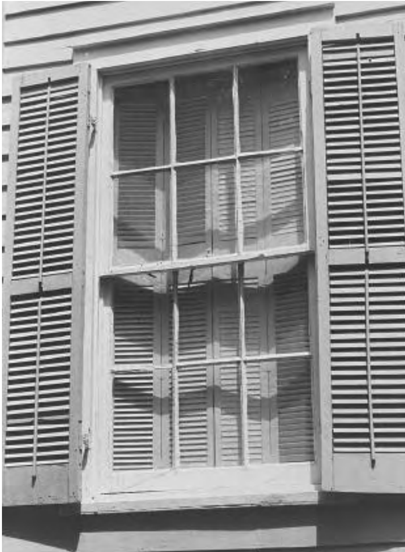
The glazing putty in this window is deteriorated in some locations. Repairs will be time consuming.
