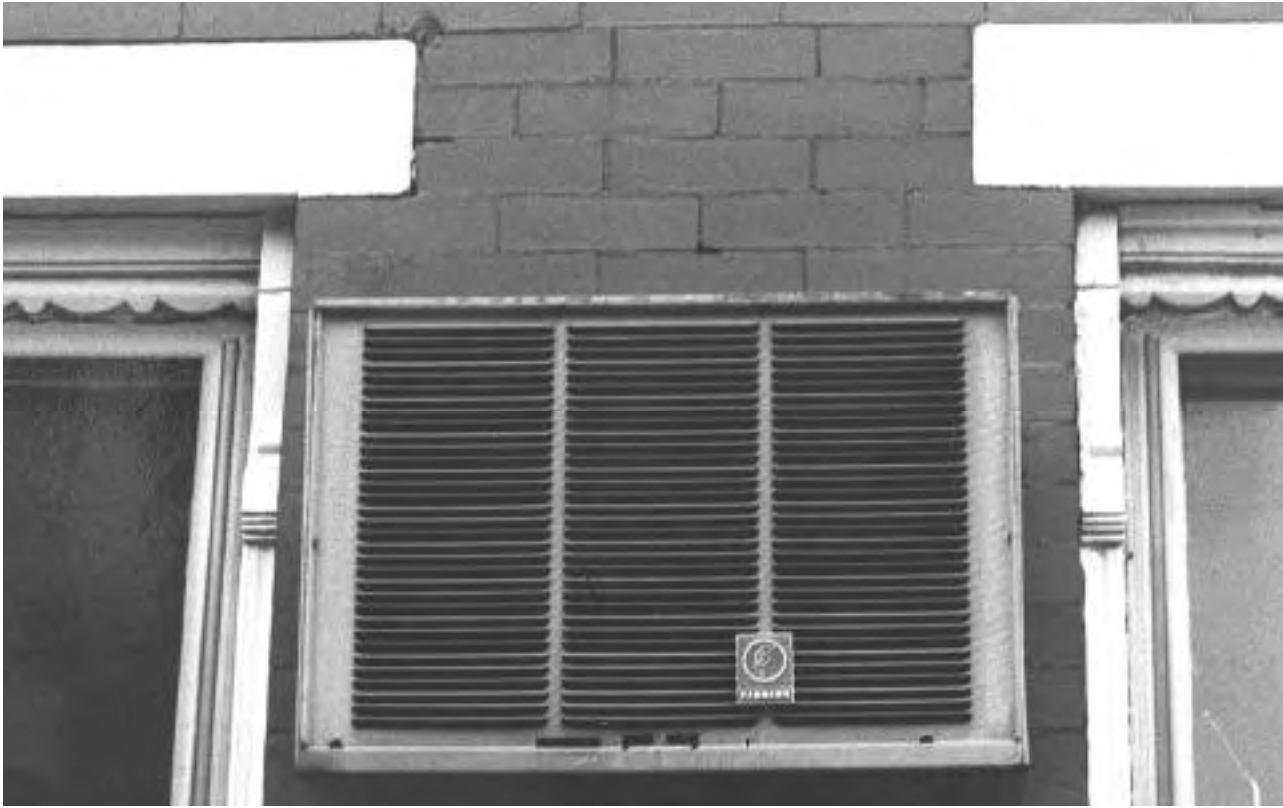
Installation of this air conditioner destroyed the structural integrity of the bearing wall between the two windows.
