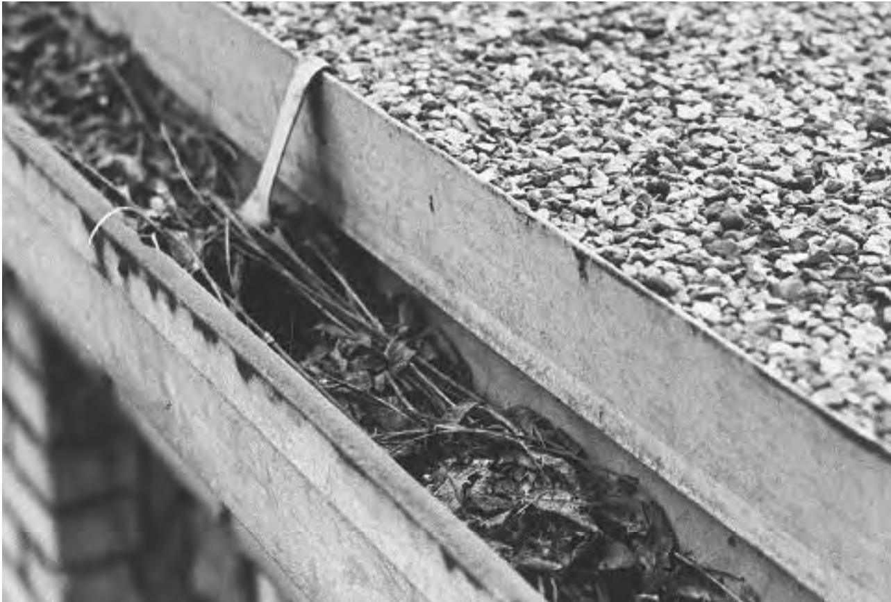
The gutters on this low-slope roof are deteriorating largely because of the accumulated detritus that they hold. They should be inspected and cleaned periodically.
