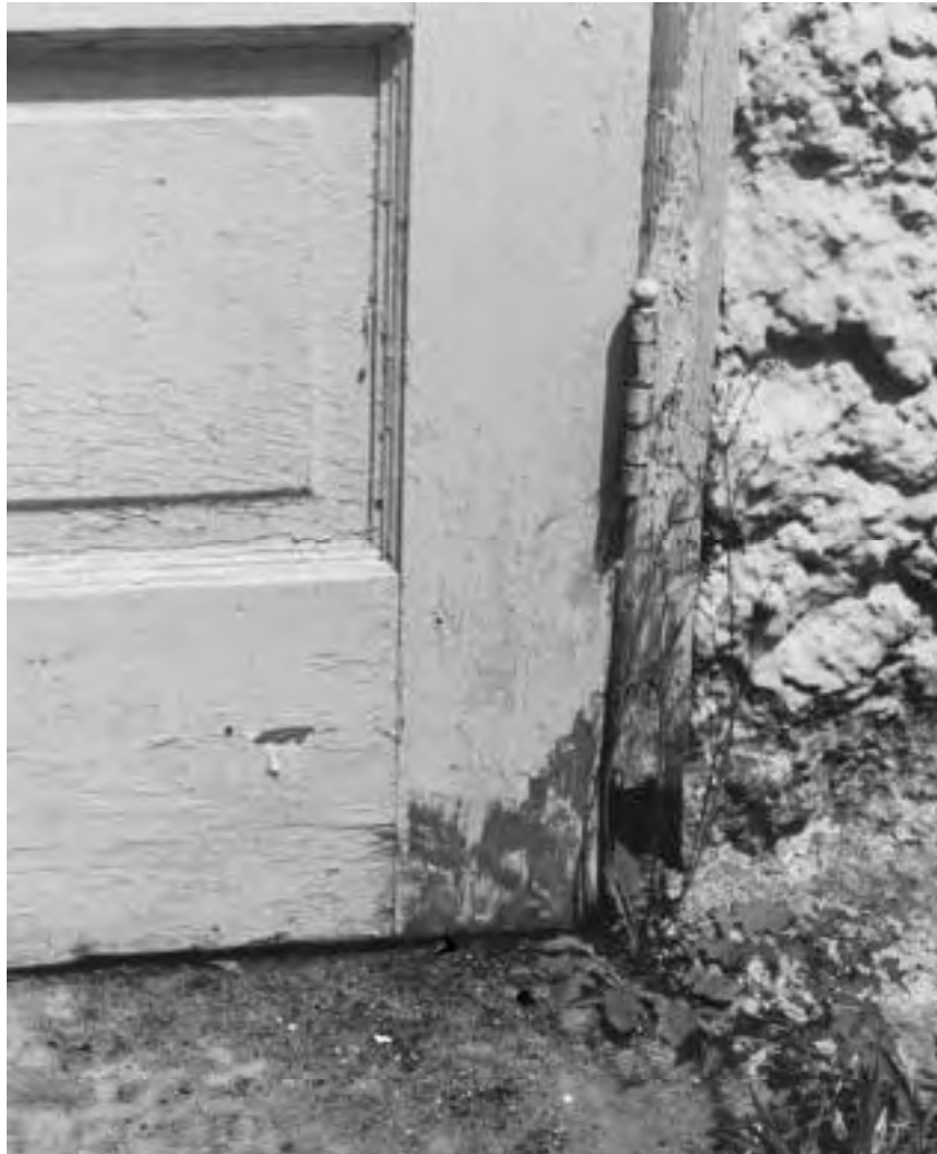
A common location of fungal and insect infestation is where wood door frames touch concrete or earth at grade.
