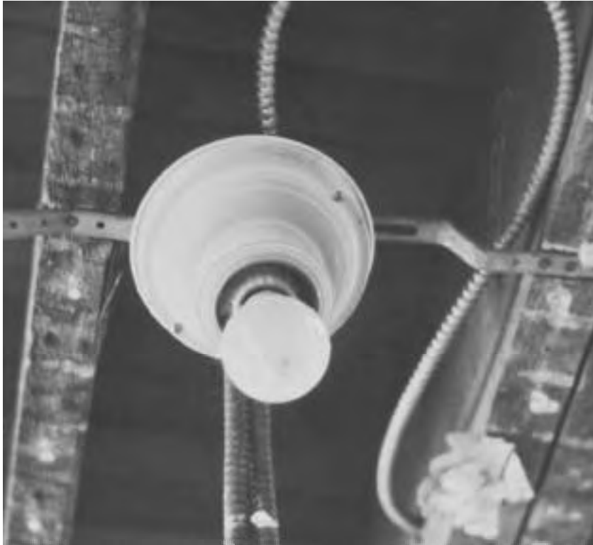
The armored cable and junction box are in good condition and can be reused, even if the lighting fixture is relocated.
