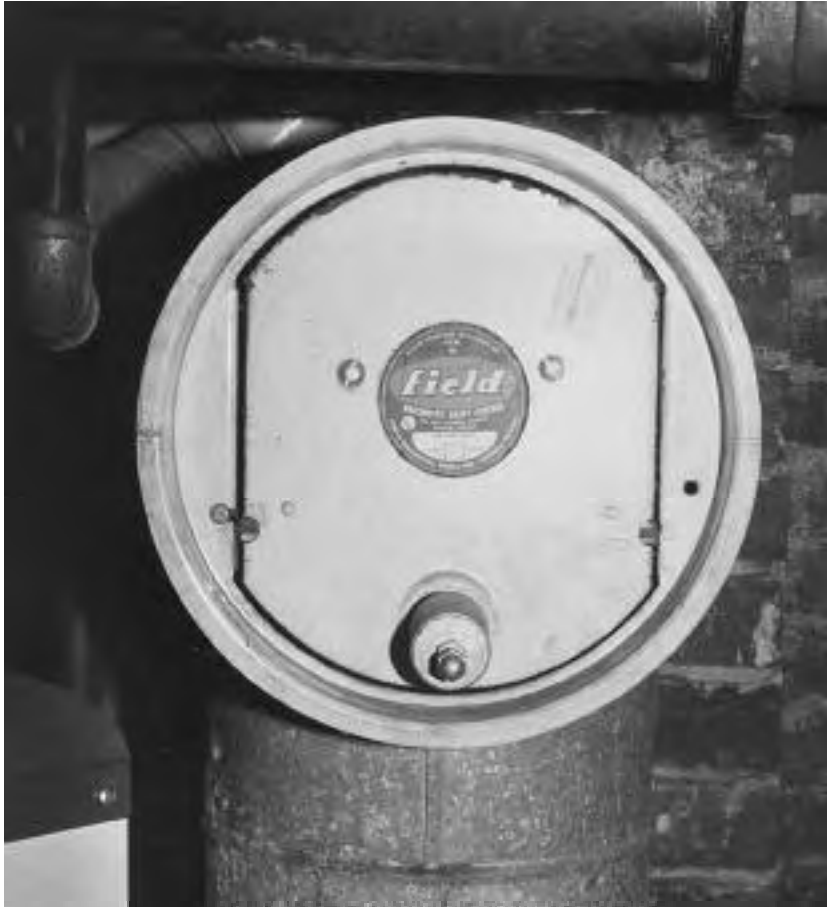
This barometric draft regulator should swing freely and open somewhat as the heating unit warms up.
