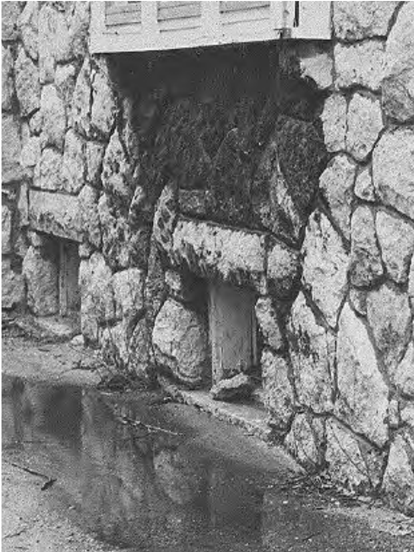
Poor site drainage leads to a variety of problems, in this case a wet basement.
