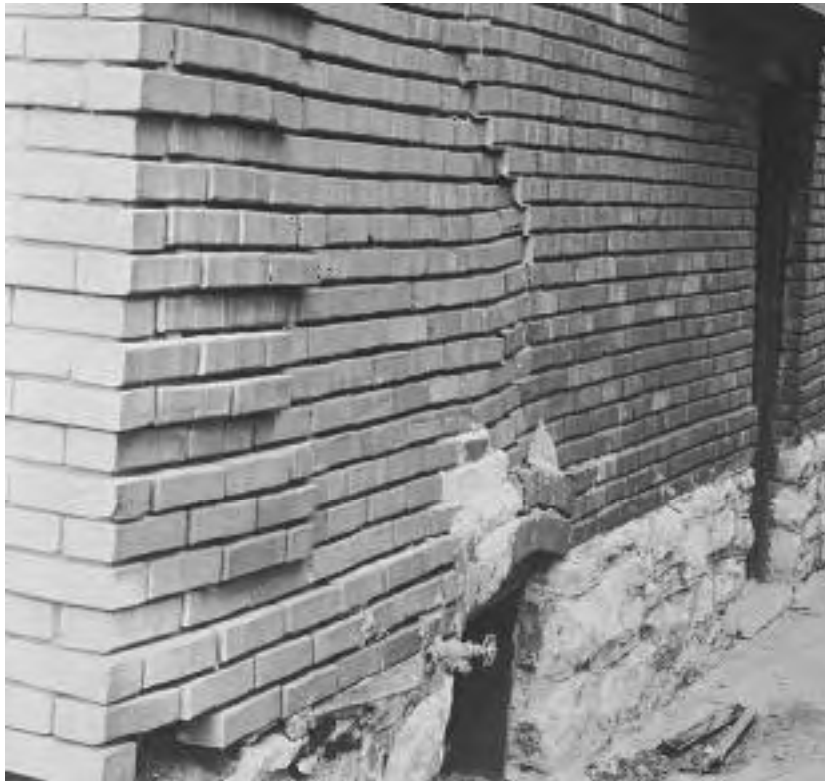
An extreme case of structural failure in a masonry wall due to foundation settlement. The wall and foundation must be completely rebuilt.
